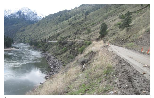
Figure 2 – Wall 8-9 area looking upstation with shallow slides right and irregular outboard
